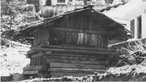
These are used to store paddy, maize, sorghum, wheat etc. Their capacity varies between 9 to 35 tonnes. The storage structure is box like made of wood and raised on pillars. Both the floor and walls are made of wooden planks whereas the thatched or tiled roof is placed over it to protect the grains from the sun or rain. The improved Kothar structure is generally made of 5 cm thick wooden planks and beams. The walls and floor are made in such a way that no gap
