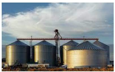
Silos/bins are classified into two groups depending upon the relative dimensions of the container. These are classified as, (1) deep bins and (2) shallow bins.
